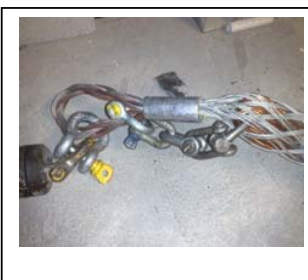
View of corrective actions, shackles attached through cable splice to pull line as secondary safety control as well as sock bolted through cable.
