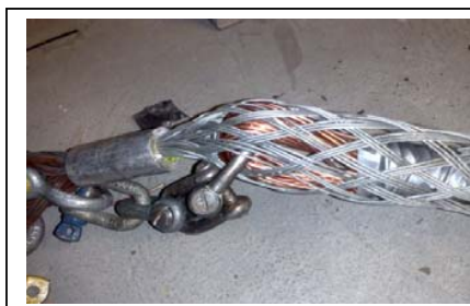
View of corrective actions, shackles attached through cable splice to pull line as secondary safety control as well as sock bolted through cable.
