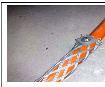
View of corrective actions, shackles attached through cable splice to pull line as secondary safety control as well as sock bolted through cable.
